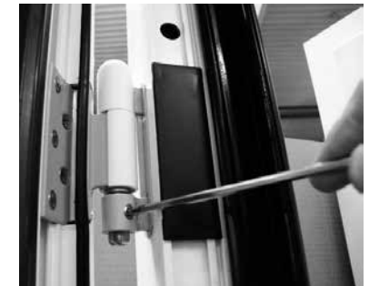
Loosen fixing screw.
