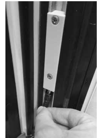
4. Insert plug into manual charging socket, close window and connect charger to socket
